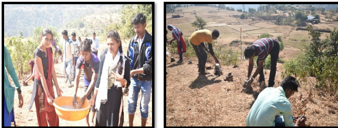
Photo No.5.8- A road was constructed in adopted village.
