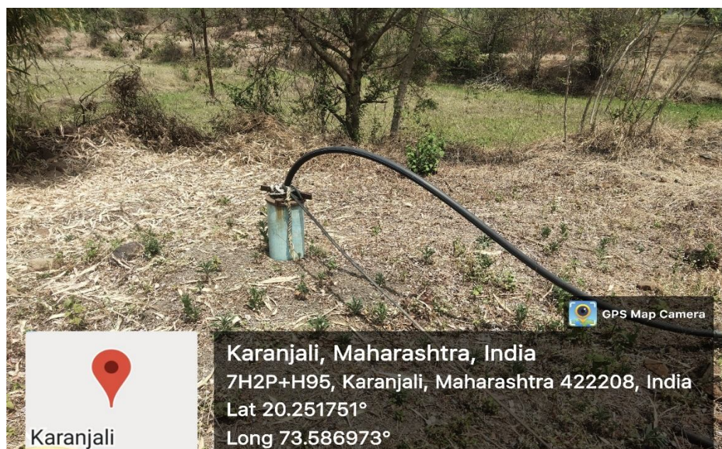
Photo No.3.1 Shows Borewell used for water supply.
