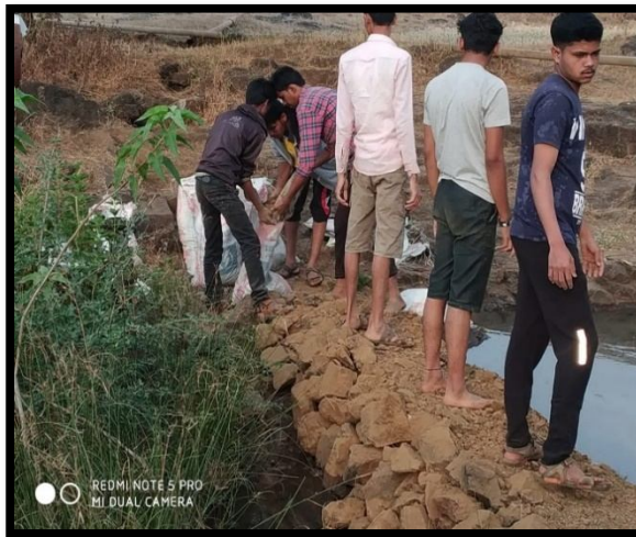
Photo No. 5.4 shows the construction of the Check Dam on the river at Devgaon Village.
